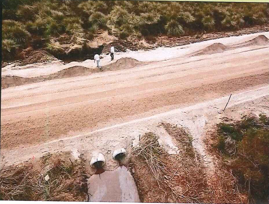
Figure 9: Construction site: Pipe-culvert at km 6.34
