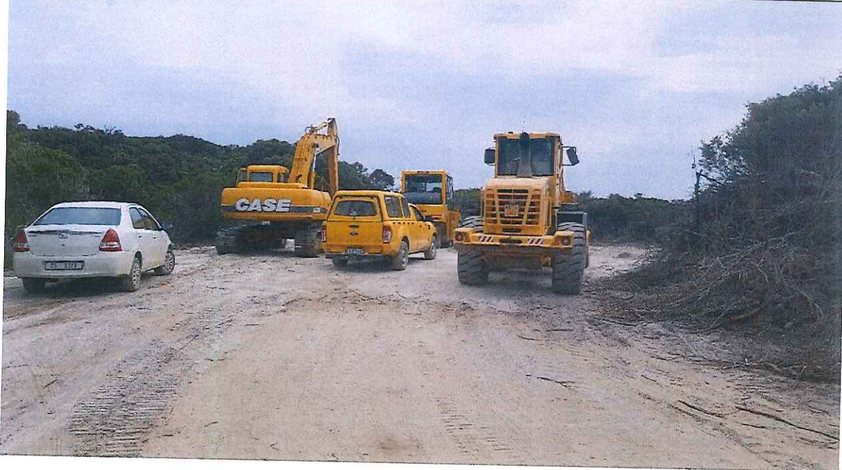
Figure 13: Construction site: Storage area for plant and equipment
