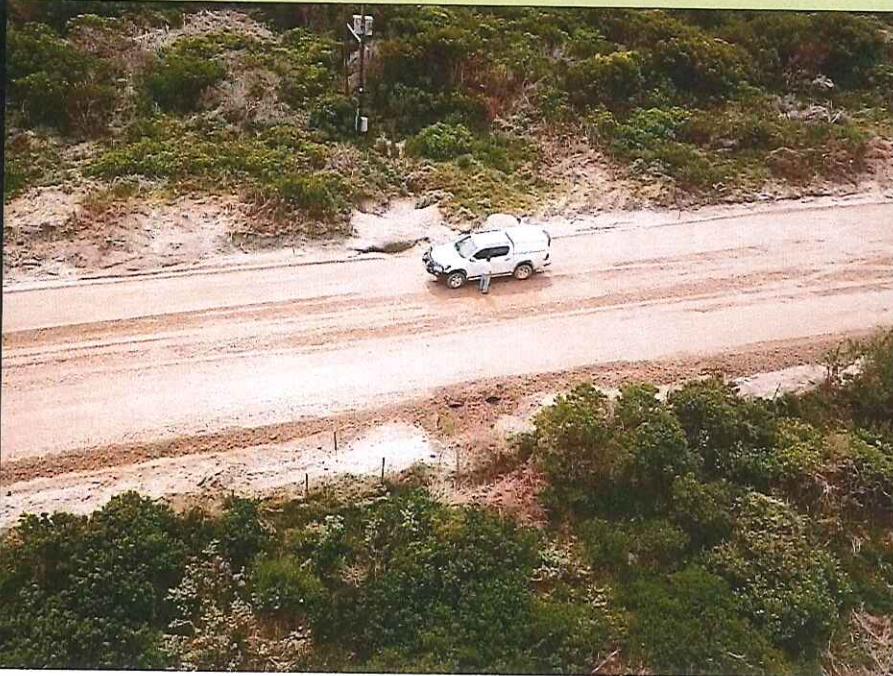
Figure 10: Construction site: Pipe-culvert at km 7.07
