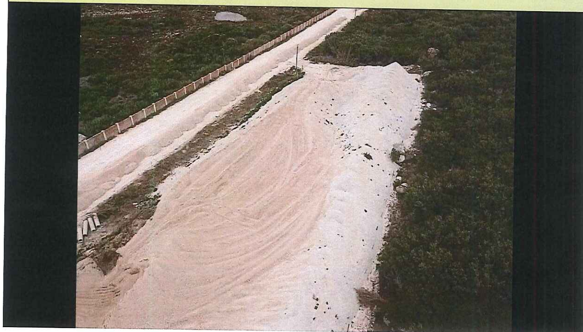
Figure 12: Construction site: Stockpile site
