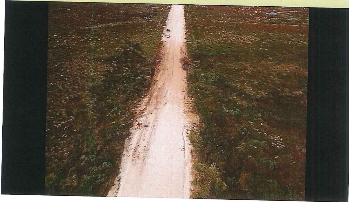
Figure 7: Construction site: Pipe-culvert at km 4.08
