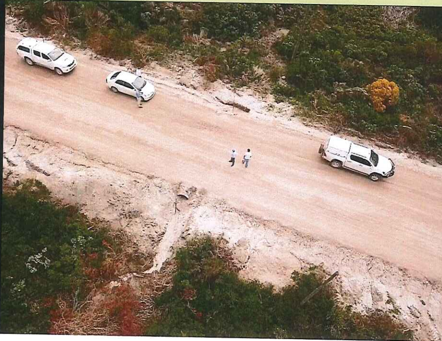
Figure 11: Construction site: Pipe-culvert at km 7.42
