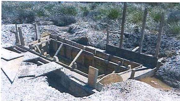
Figure 10: Construction of new culvert inlet
