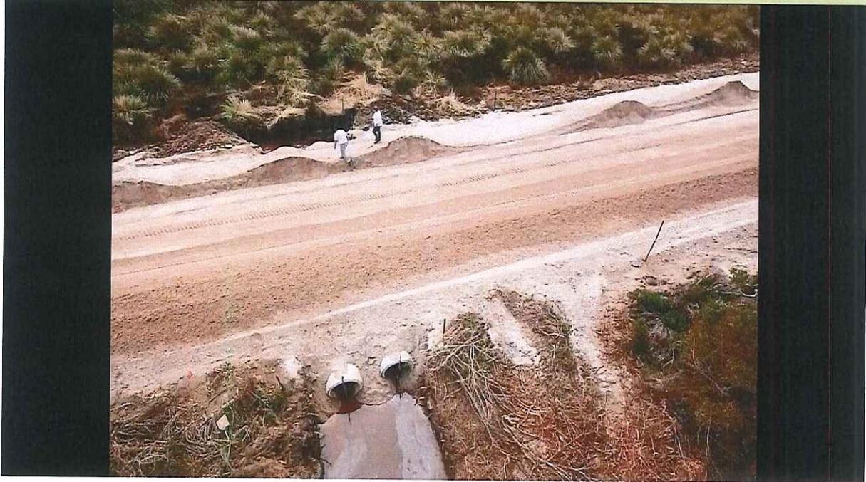
Figure 7: Construction site: Pipe-culvert at km 6.34
