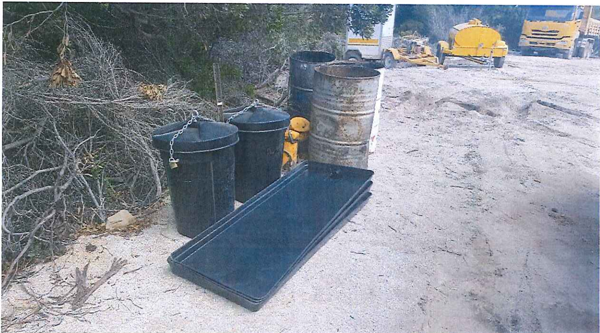
Figure 11: Construction site: Drip trays and refuse bins
