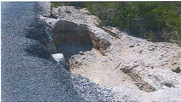
Figure 8: Excavation of culvert at km 7.07
