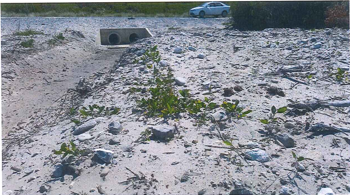
Figure 7: Drainage channel at culvert at km 6.34 outlet
