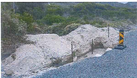
Figure 9: Excavation of culvert at km 7.42
