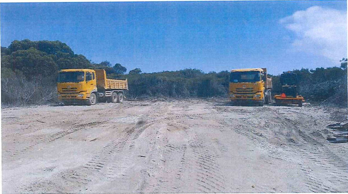
Figure 12: Construction site: Storage area for plant and equipment
